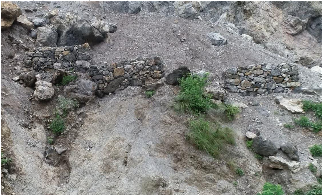
Photograph 8- Retaining structures provided near the mining site
