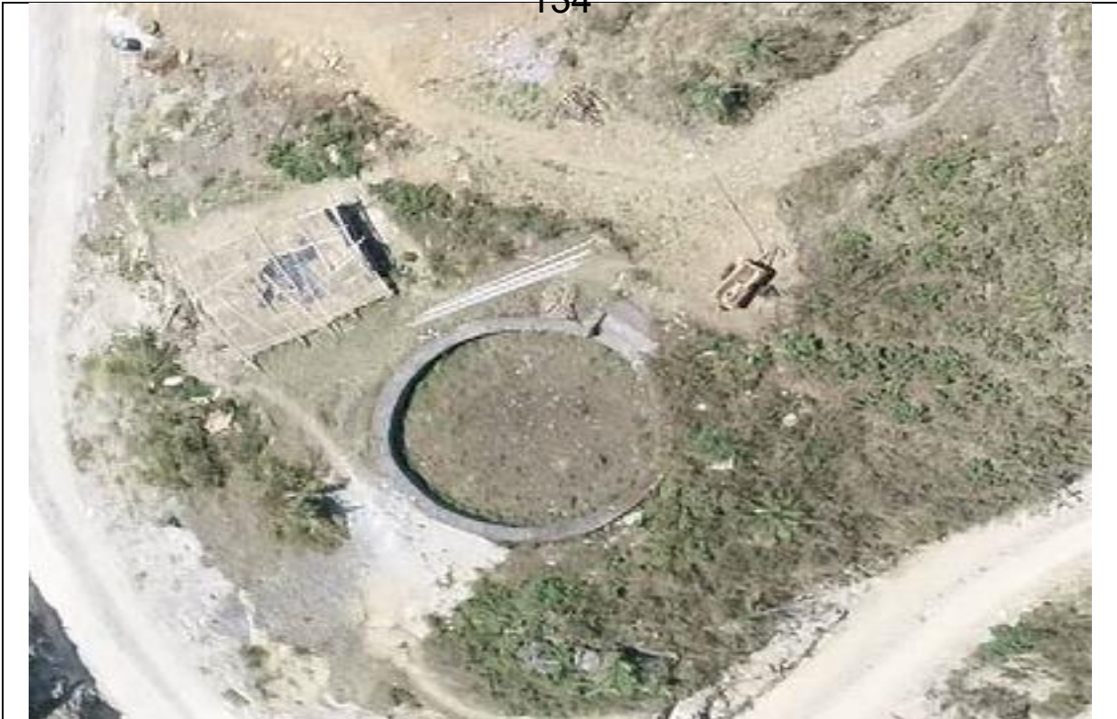
Photograph 3- Water harvesting tank
