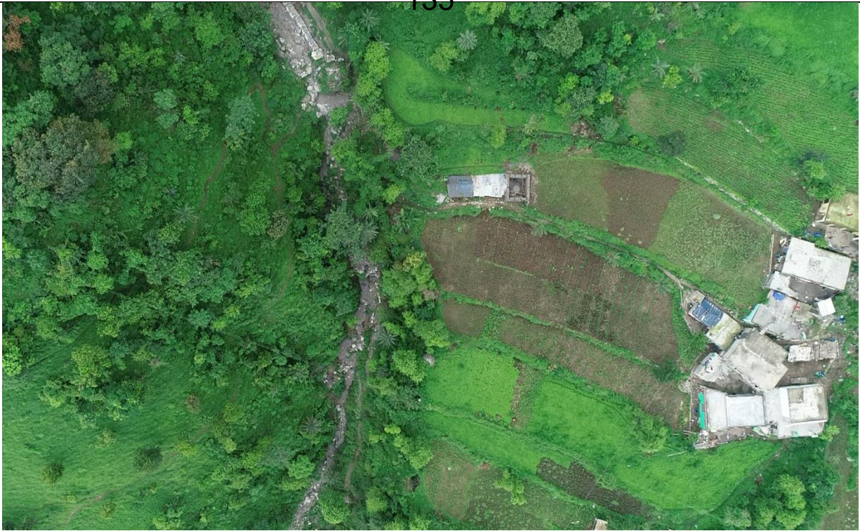
Photograph 5 – Retaining structure provided at the channel of nallah flowing nearby village and no debris observed in agricultural fields or damage to property of villagers
