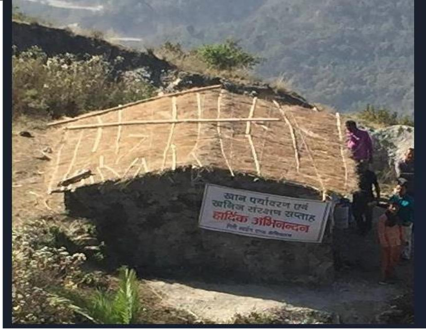
Photograph 1- Rest shelter for labour
