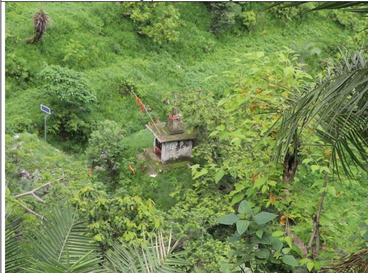
Photograph 4- Village Temple intact and no damage to the temple due to debris as alleged
