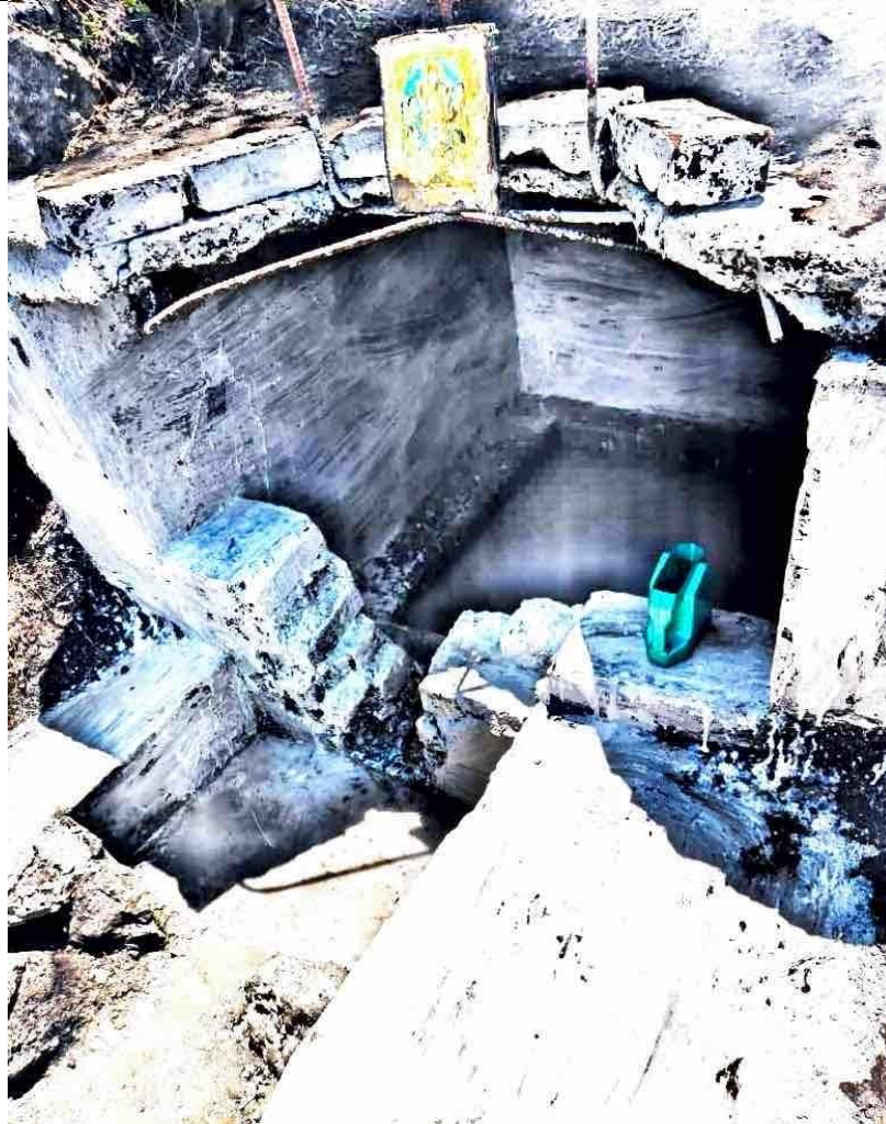
Photograph 2- Restoration of bawri (potable water resource)
